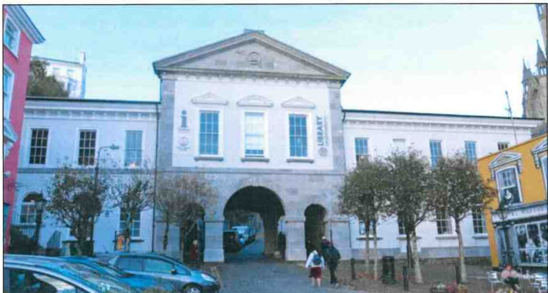
• Fig 10. Arch fronted road crossing under building from Casement Square.
