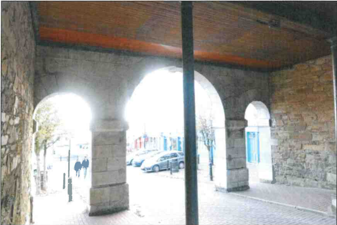
• Fig 15. Building undercroft looking South.
