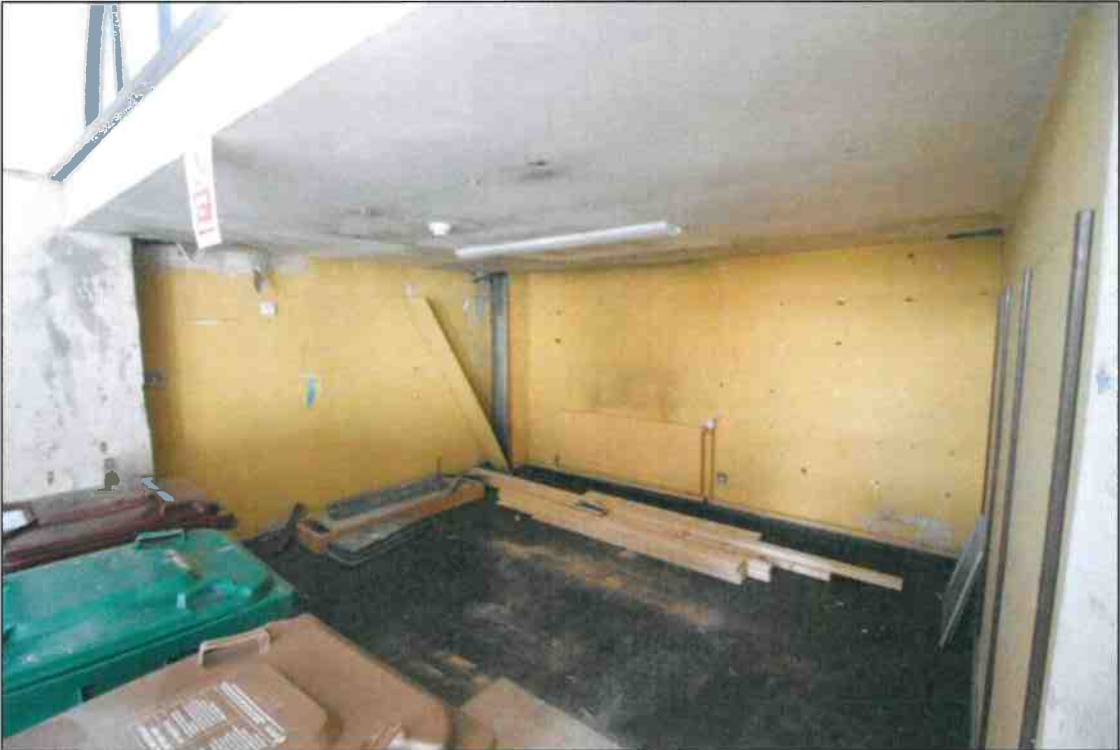
• Fig 63. Room 10. Rear flat North roofed rooms.
