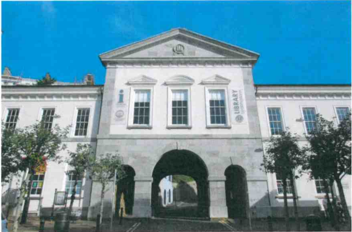
• Fig 2. South Elevation and view up 'West View' road.
