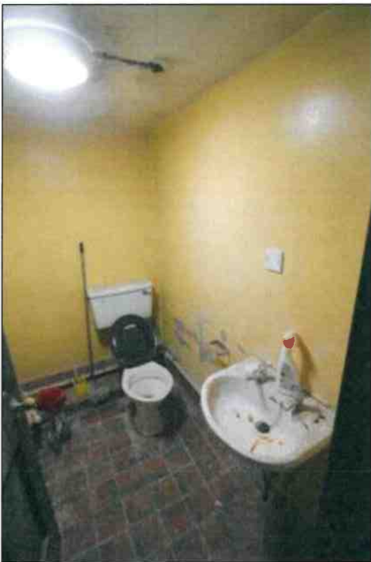
• Fig 68. Toilets off room 11 .
