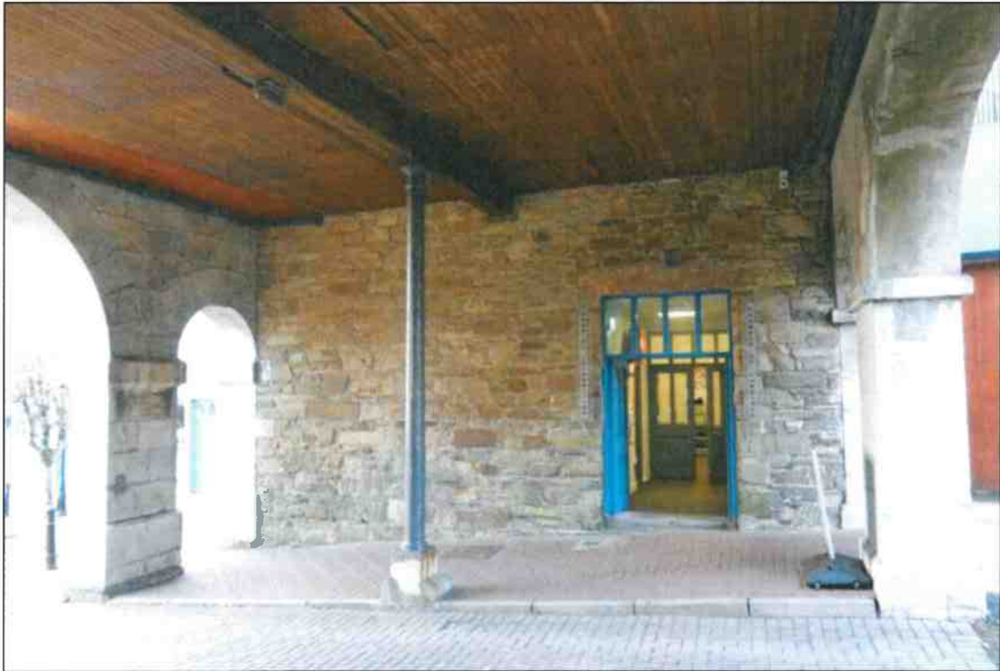
• Fig 16. Building undercroft looking West towards Tourist office.
