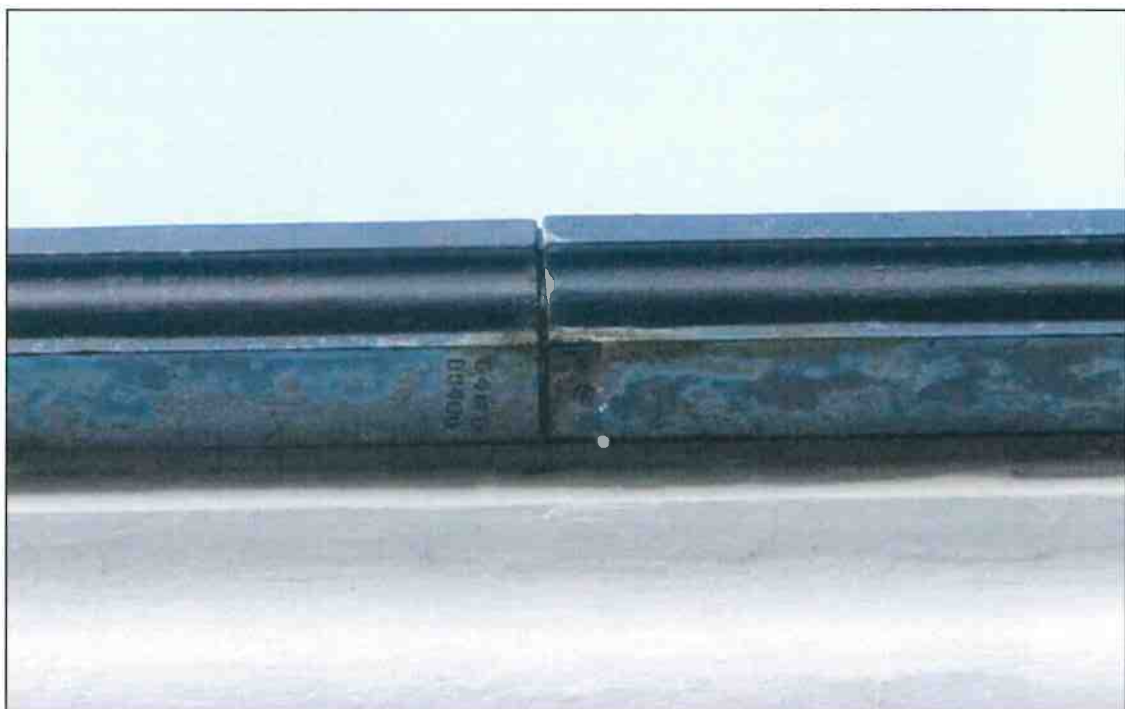
• Fig 78. Leaking gutter junctions in places (over Eastern wing South elevation.) Corrosion evident also.
