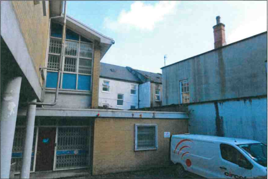
• Fig 20. North elevation looking East through EIR car park.
