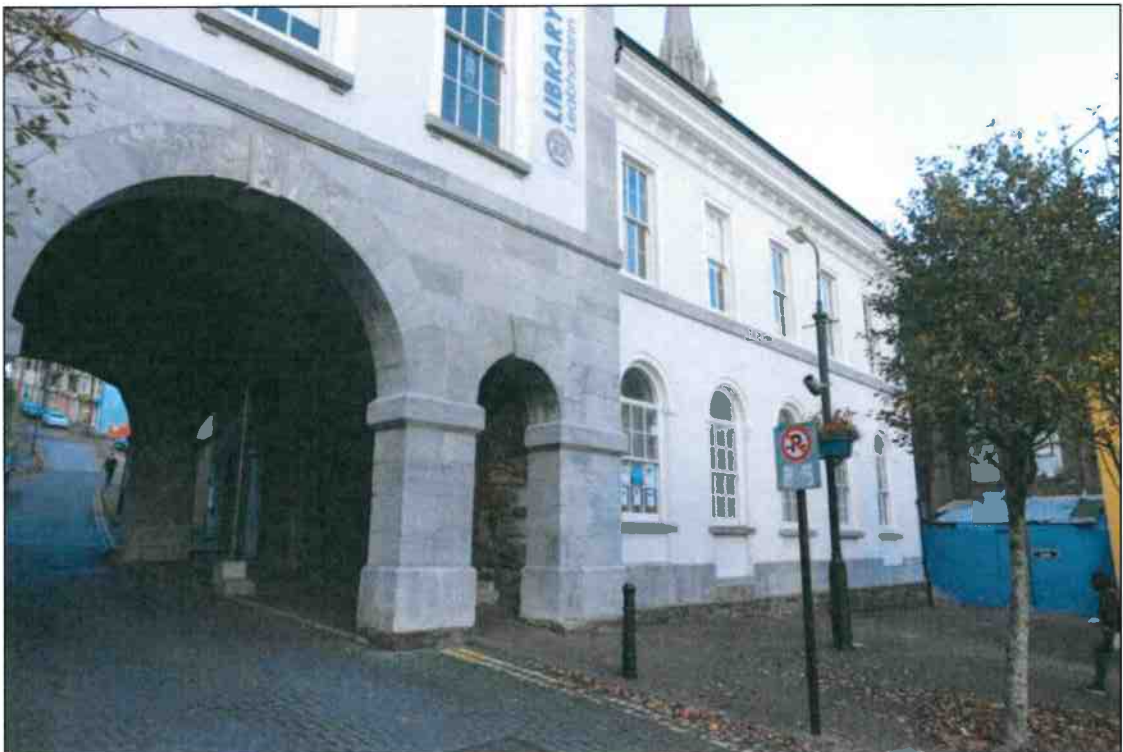
• Fig 12. South elevation and East wing, now housing library on upper level and site for new Hub below.
