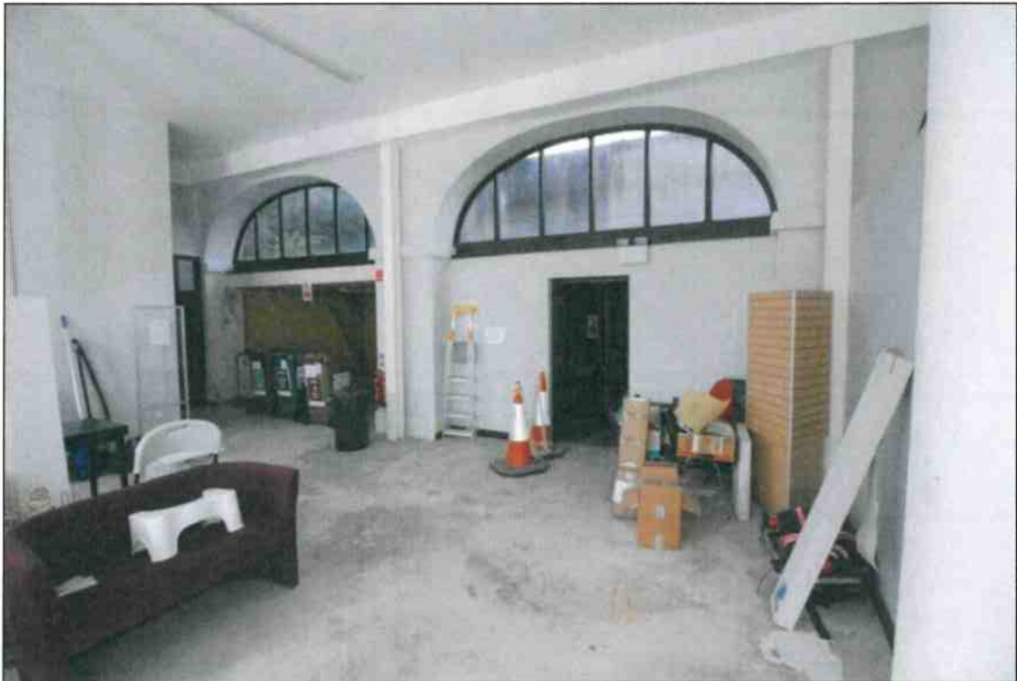
• Fig 60. Room 9. Rear flat North roofed rooms under arches.
