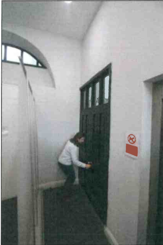
• Fig 66 Entrance to plant room.
