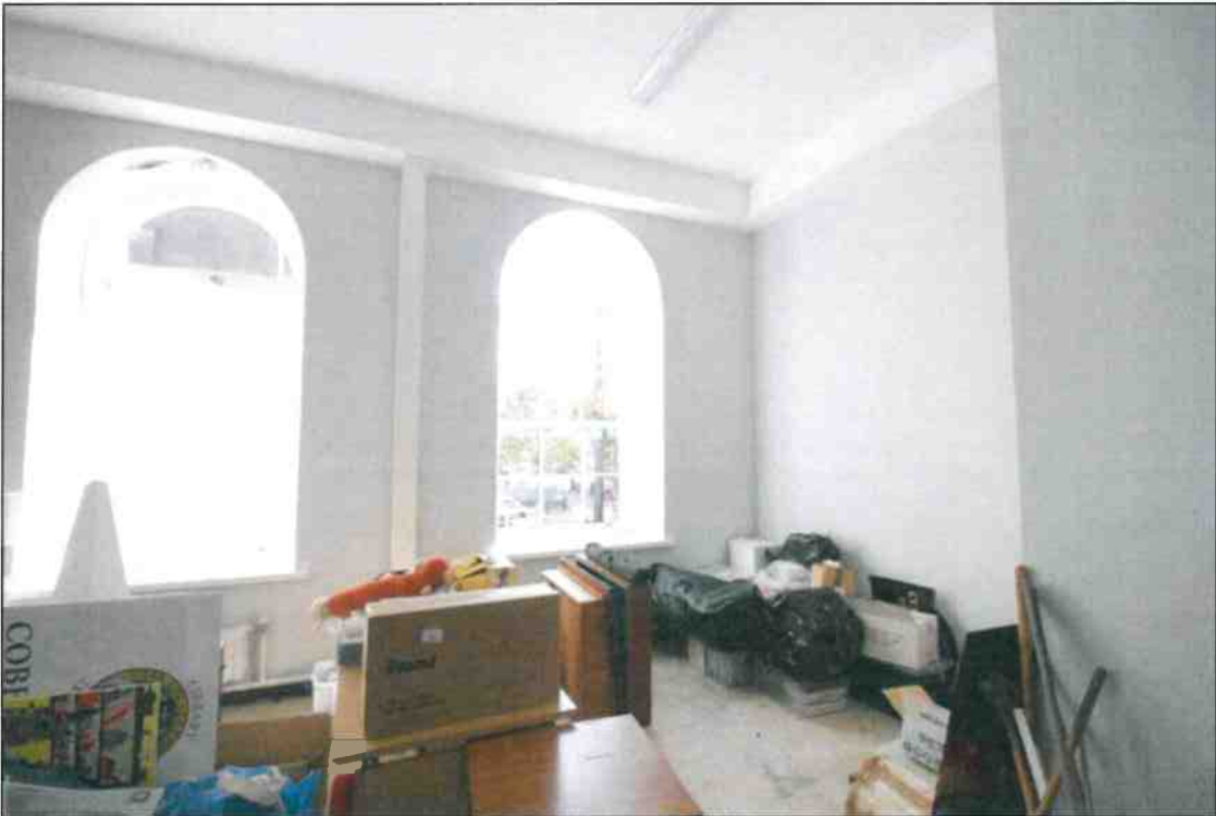
• Fig 64. Room 9. Looking South.
