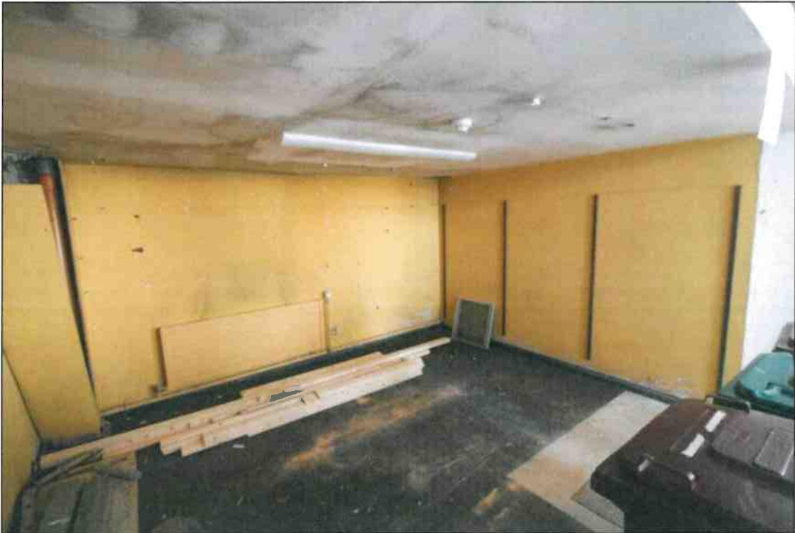
• Fig 62. Room 10. Rear flat North roofed rooms.
