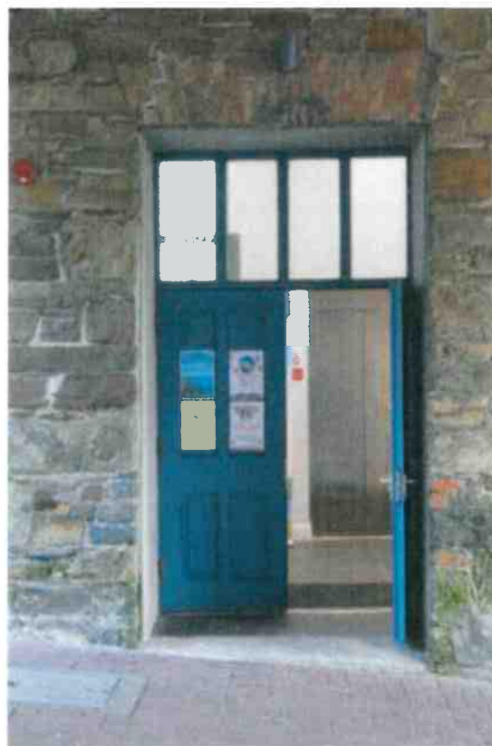
• Fig. 85. Library ramped entry step.
