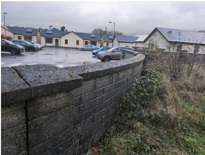
Plate 4. Concrete block wall along northern boundary
