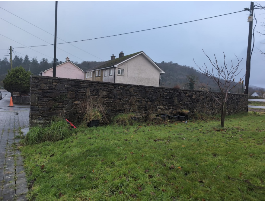
Plate 6. Stone wall at south of site
