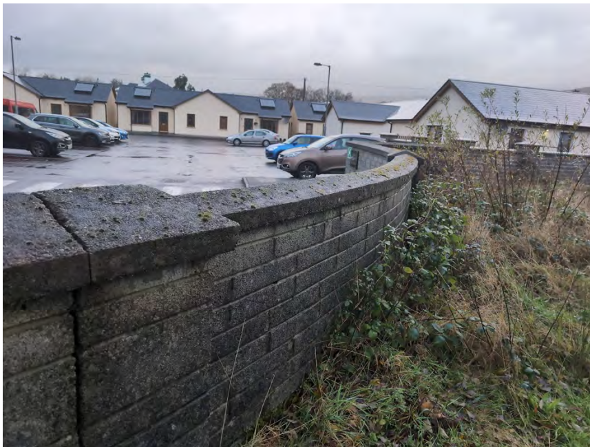
Plate 4. Concrete block wall along northern boundary
