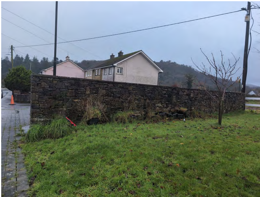
Plate 6. Stone wall at south of site
