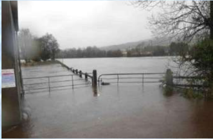
Flooding at Ballymakeera Bridge October 2011
