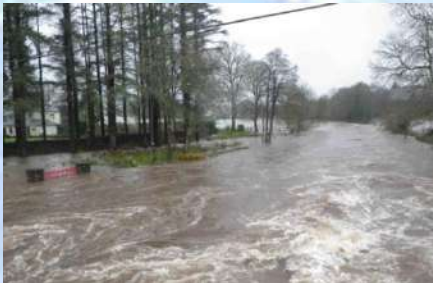
Flooding at Ballyvourney Bridge October 2011
