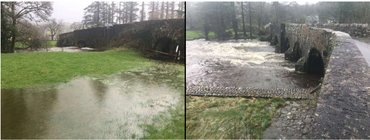
Figure 1 Ballyvourney Bridge (upstream and downstream)
