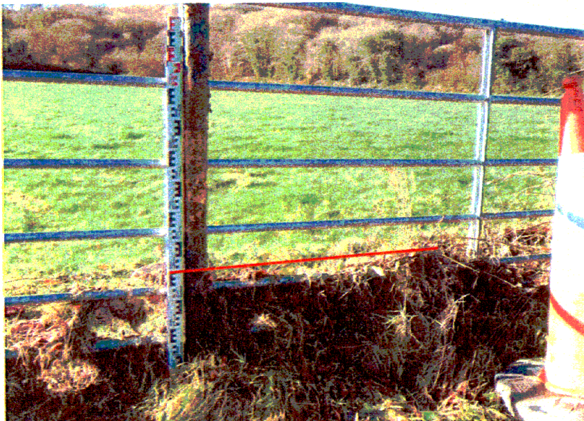
Photo 2 Trash level on gate downstream of Baile Mhic Íre Bridge (NGR 121300 76313)
