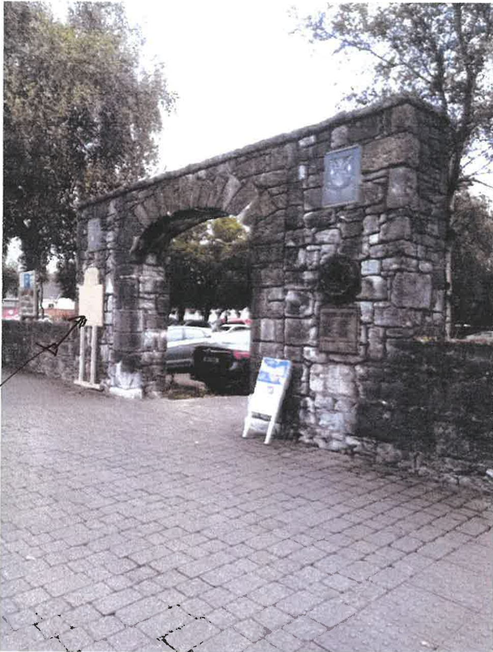
Location Br Wall.
