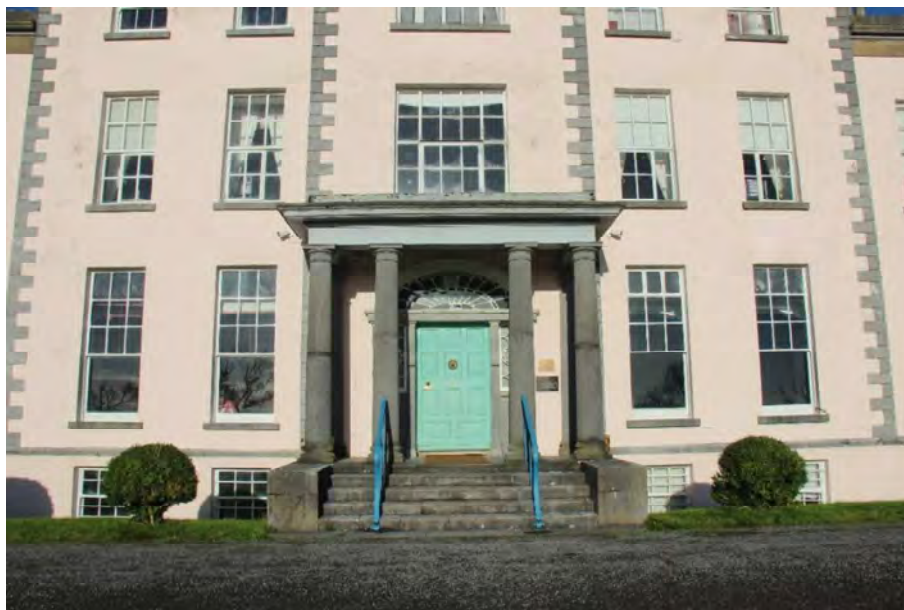
Photograph 1 - Longueville House Front Entrance
