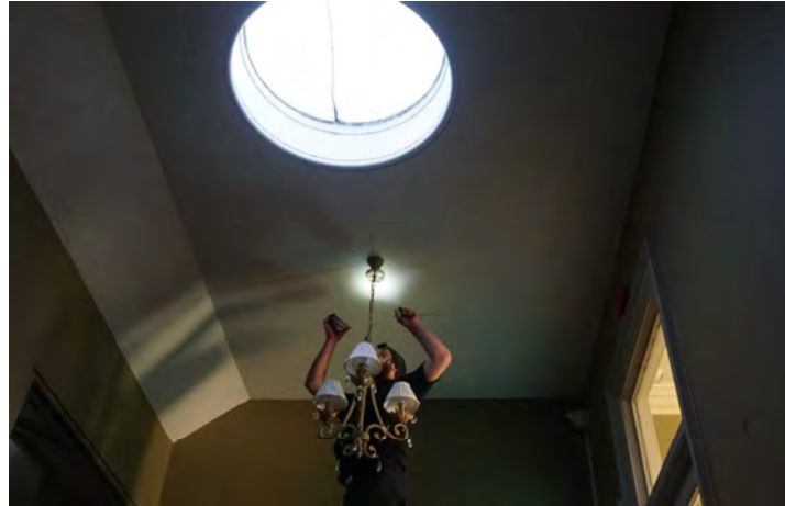
Figure 8 Using existing openings in the ceiling
