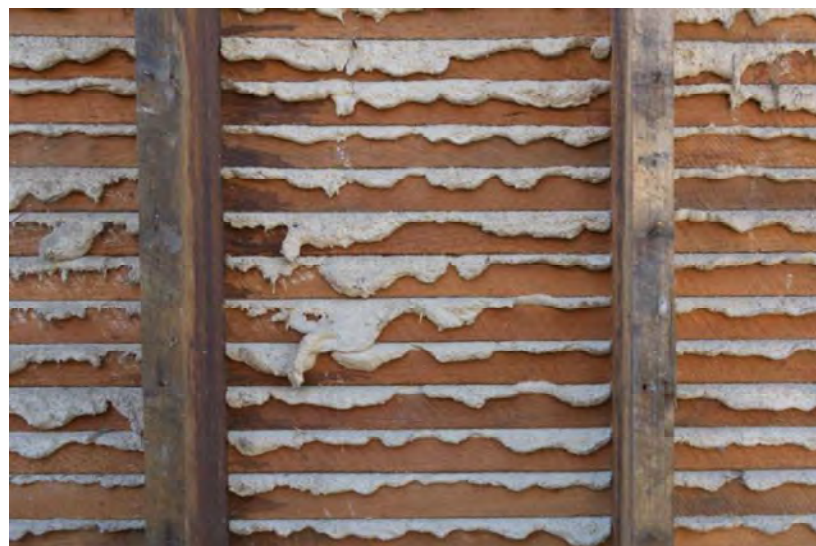
Figure 7 Upper surface of Lath and Plaster ceilings https://cdn.britannica.com/64/132064-050-A7A9675C/laths-base-plaster.jpg
