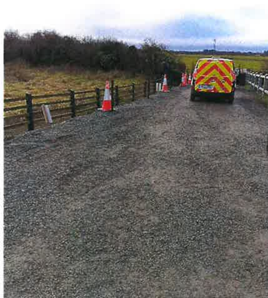
Figure 11: Crushed Rock Roadway
