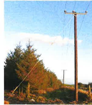
VIEW OF LIGHT ANGLE POLE (LAP)
