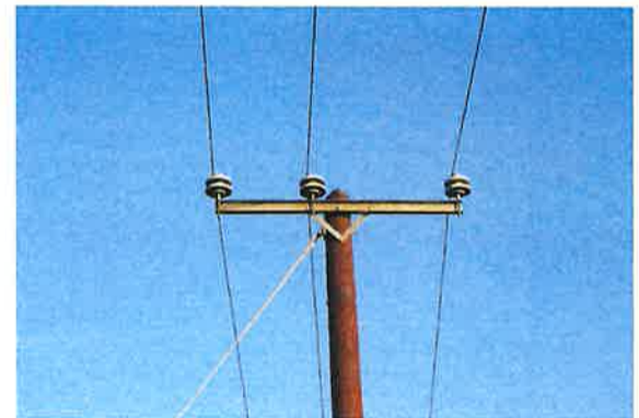
VIEW OF LIGHT ANGLE POLE HEAD
