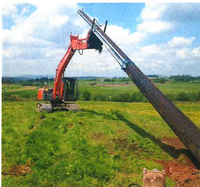
Figure 8: Installation of Wood Polesets
