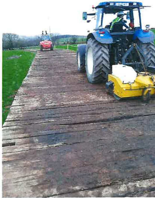
Figure 10: Timber Roadway (Bog Matt)
