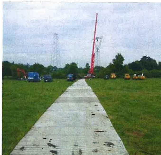
Figure 9: Temporary Aluminium Panel Tracks
